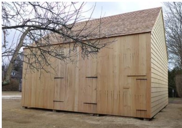
The north side of the finished barn is sheathed with wide vertical planks of white pine. Mark Segal
